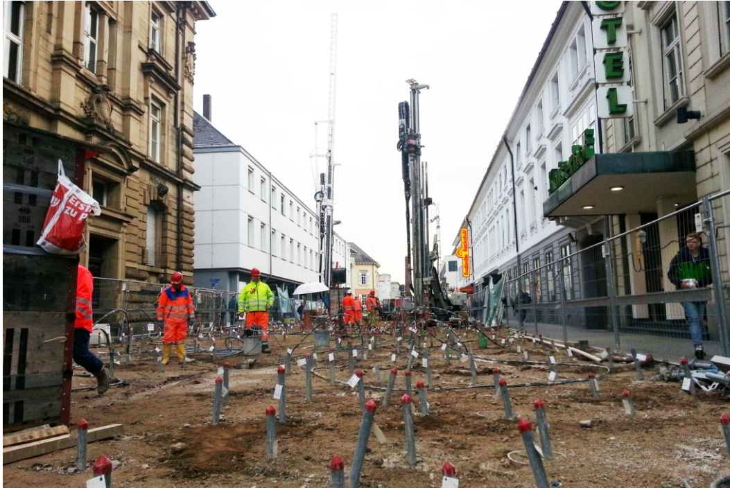
Drilling and grouting works in the Karl-Friedrich-Street
